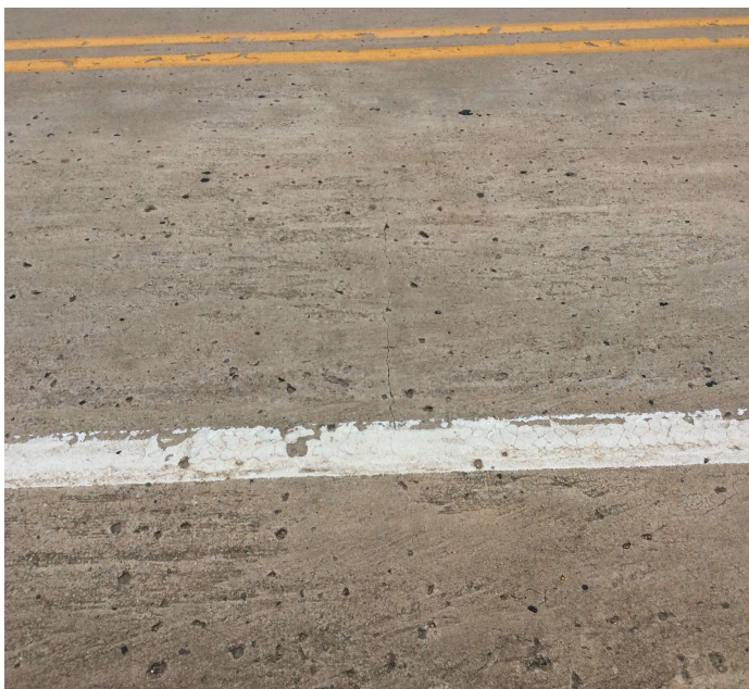
PHOTO 4 Description Typ. Cracking in Deck.
