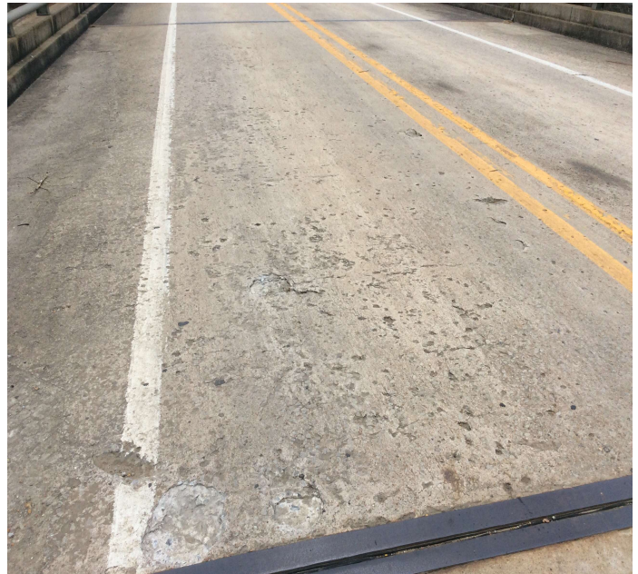
PHOTO 2 Description Typ. Delam, Cracking, Scaling & Spalling in Deck.
