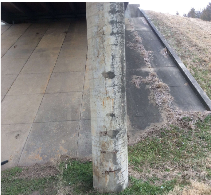
PHOTO 1 Description Delam, Cracking, Scaling & Spalling W / Rebar Exposed in Column 2 at Pier 4.
