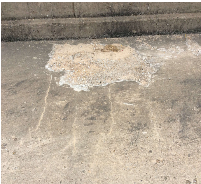
PHOTO 3 Description Cracking & Scaling in Gutters.
