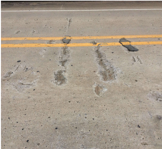
PHOTO 1 Description Typ. Delam, Cracking, Scaling & Spalling W / Rebar Exposed in Deck. Mainly in Span 3.
