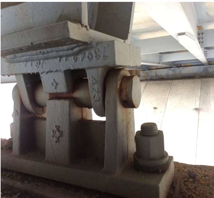
PHOTO 1 Description Shear key missing from Rt. Side of bearing pin at bearing 4 Ahd. Side pier 4.
