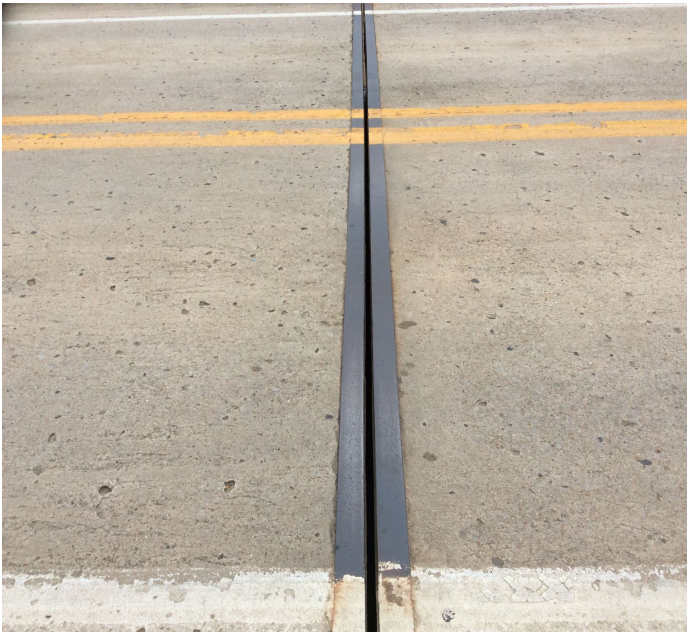
PHOTO 1 Description Seals Missing at Joints.
